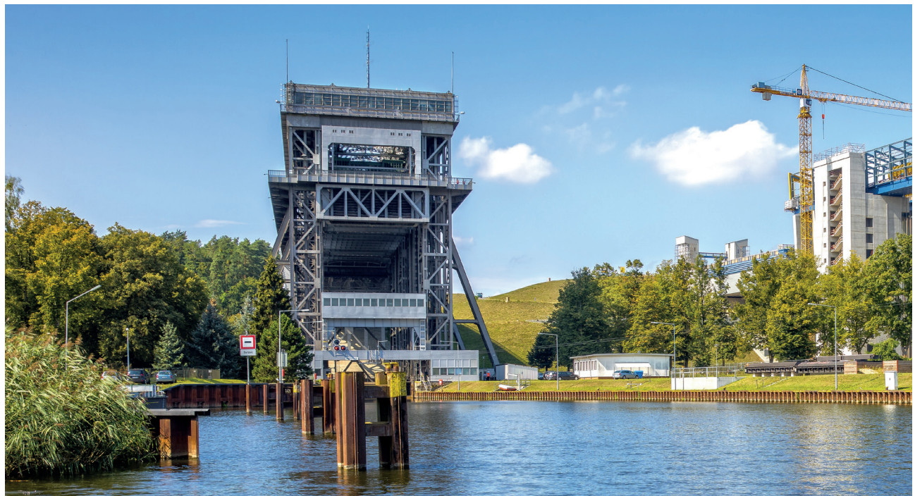
On the left is the old ship lift, which will support the new lift on the right for some time after its opening.
