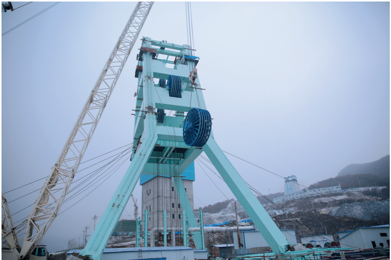
Fig. 1: Start of installation on site with the fitting of rope sheaves in the winding head of the Sishanling mine. Copyright 2022 Tianjin SIEMAG TECBERG.
