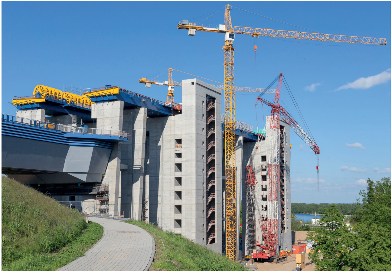
The terrain level to be overcome at the new ship lift is 36 m.
