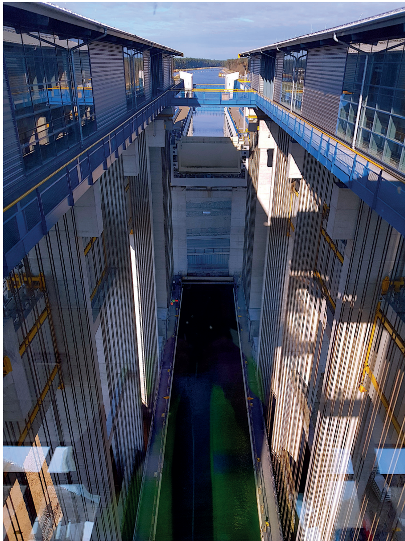
View of the trough with the steel cables as connection between trough and counterweights.
