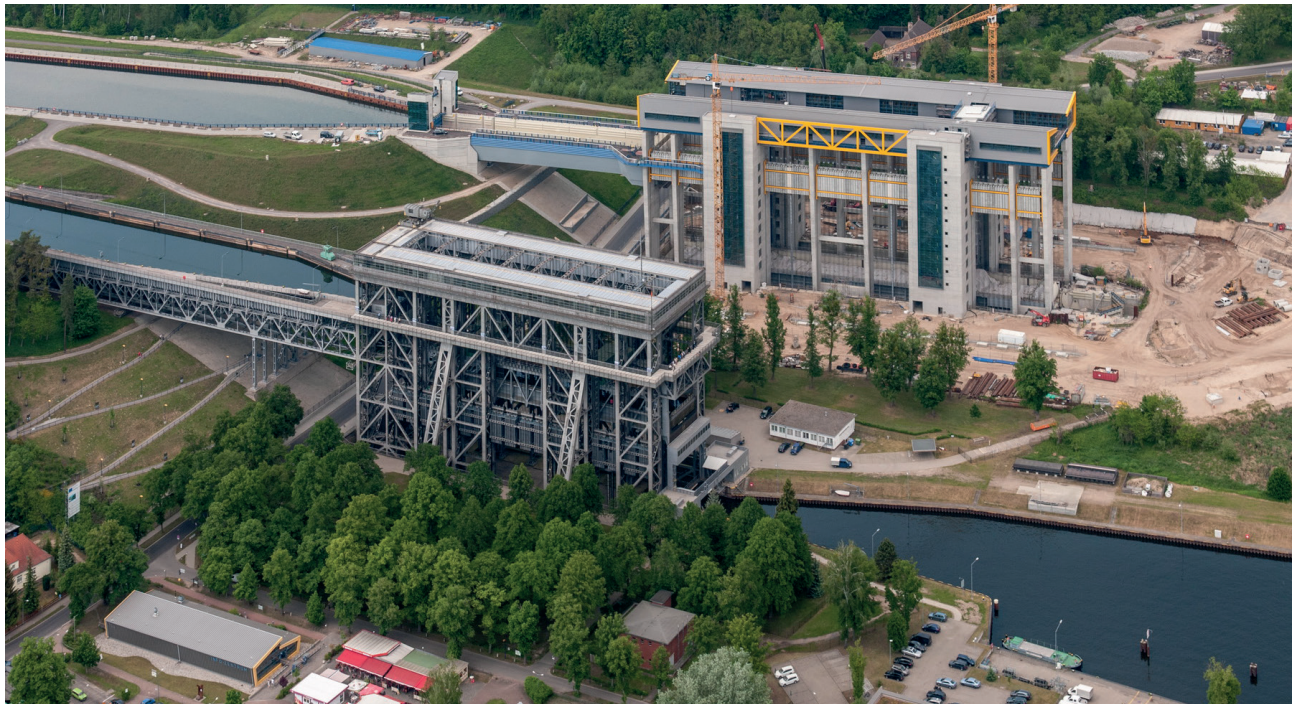
In the foreground the old ship lift, which will support the new lift in the background - here in the construction phase - for a while yet. (Photo Copyright Ralf Roletschek / Roletschek.at)
