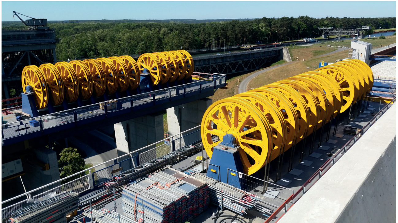
View of a part of the total of 112 installed double rope sheaves. In the background left the old ship lift.
