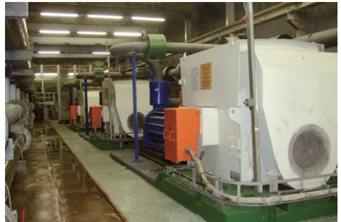
High-pressure pumps with driving power of approx. 3 x 2,500 kW, level -1,200 m/level -2,400 m
