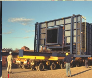
Unloading station arriving on site
