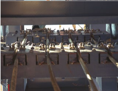
CLD in operation
