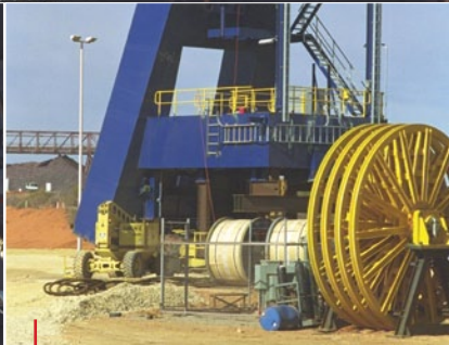
Pre-assembled sheaves and upper headframe
