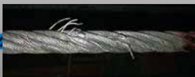
Wire break with protruding wire pieces
